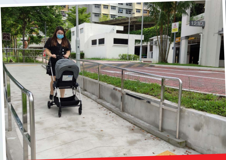
BFA Ramp near 121D Canberra Street
