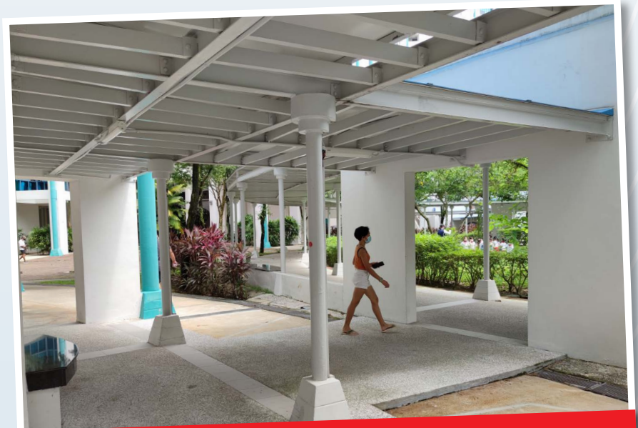
Upgrading of Covered Linkway from Blk 468B Admiralty Drive to Circular Linkway
