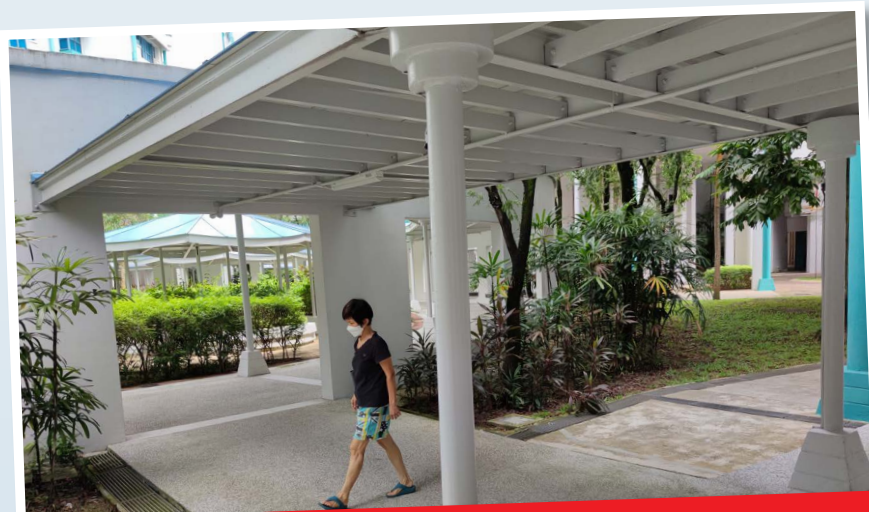
Upgrading of Covered Linkway from Blk 468C Admiralty Drive to Circular Linkway
