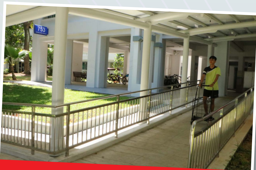
Construction of Ramp near Blk 753 Woodlands Circle
